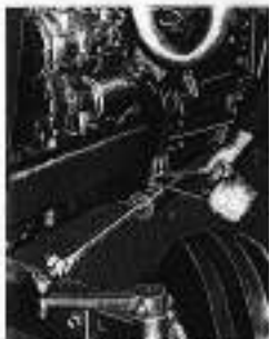
Fig. 12 - Bleeding the steering system
